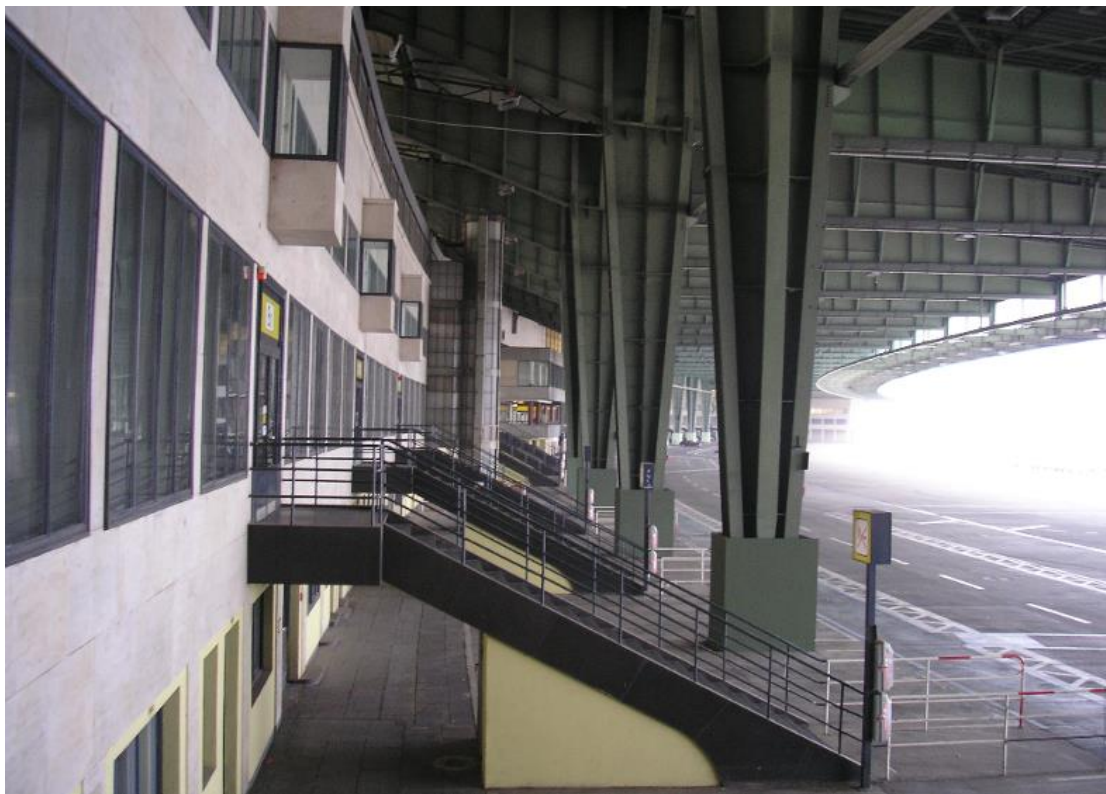
Figure 5. Tempelhof airport: the steel roof of the building boldly stretching along the outer side of the semi-circular building (Photograph taken by author)
