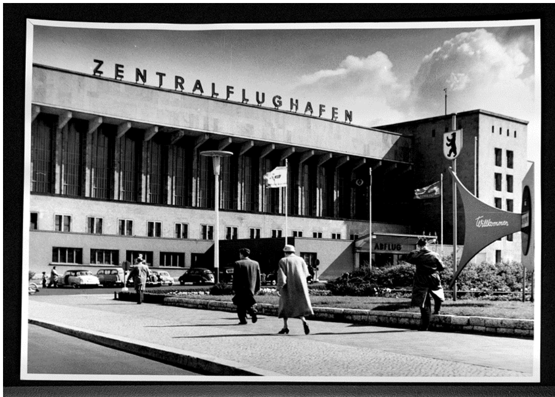
Figure 3. Tempelhof airport: post-war operation (DHM, BA 97/2356)
